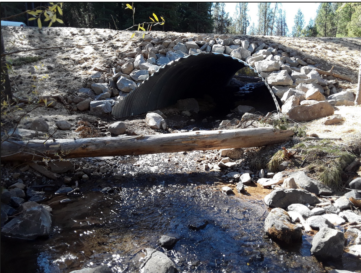
Deer Creek Culvert Replacement After
