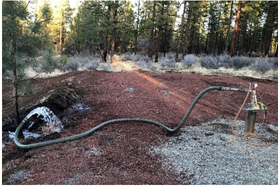
Photo 5: Well Testing, near Proctor Creek
