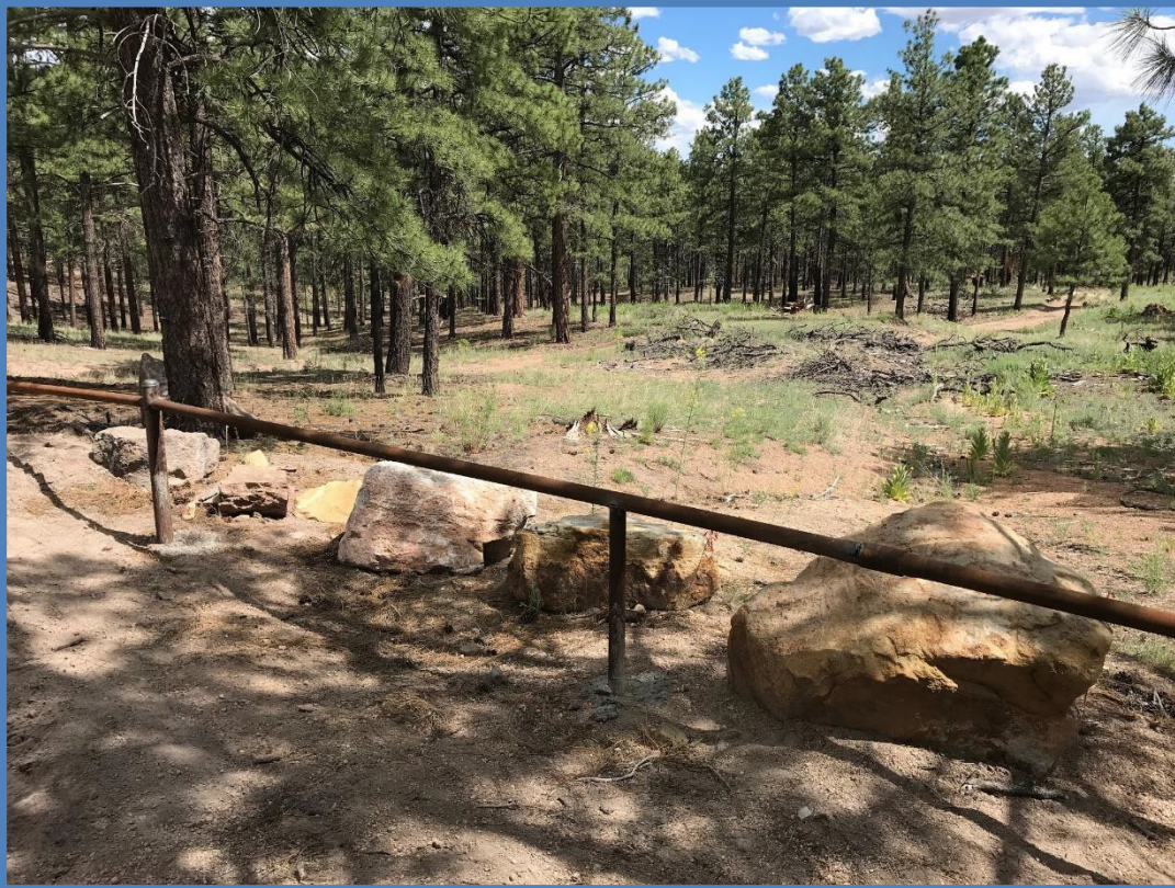
Pipe barrier installed to prevent vehicle access to a pueblo ruin. July 2019
