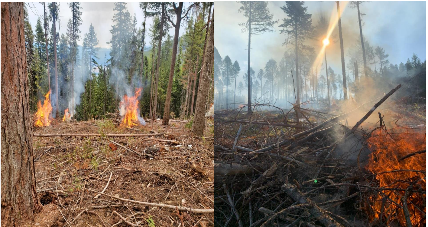
Figure 5: East Fork Stew Timber Sale Unit 4 - Purchaser grapple piling, and Forest Service pile burning.
