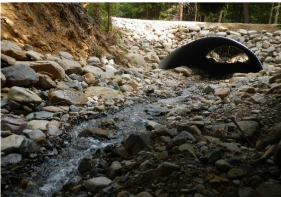
Completed bottomless arch— looking downstream
