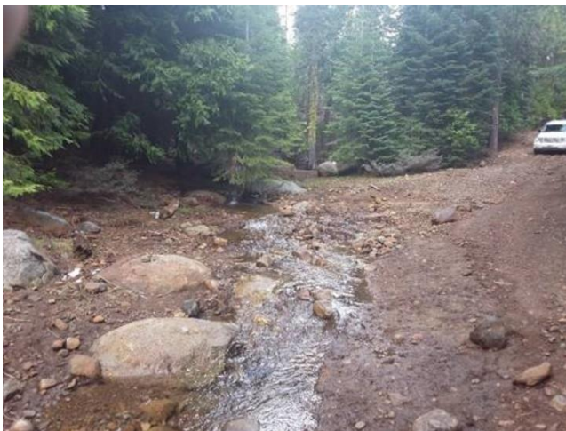
An example of culvert work needed in the Power Fire area: Channel created along the road due to plugged culvert (left) and culvert downstream (right). Photo by Joe Chow
