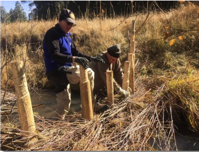
Volunteers constructing beaver dam analogs on the Rio Cebolla, October 2017; and a functioning structure
