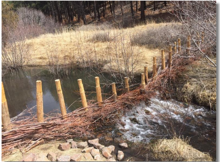
Volunteers constructing beaver dam analogs on the Rio Cebolla, October 2017; and a functioning structure
