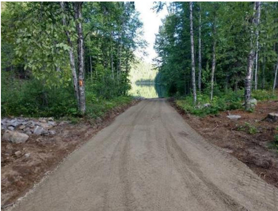
Figure 8: Boat launch reconstructed to reduce sediment flow into Solomon Lake.
