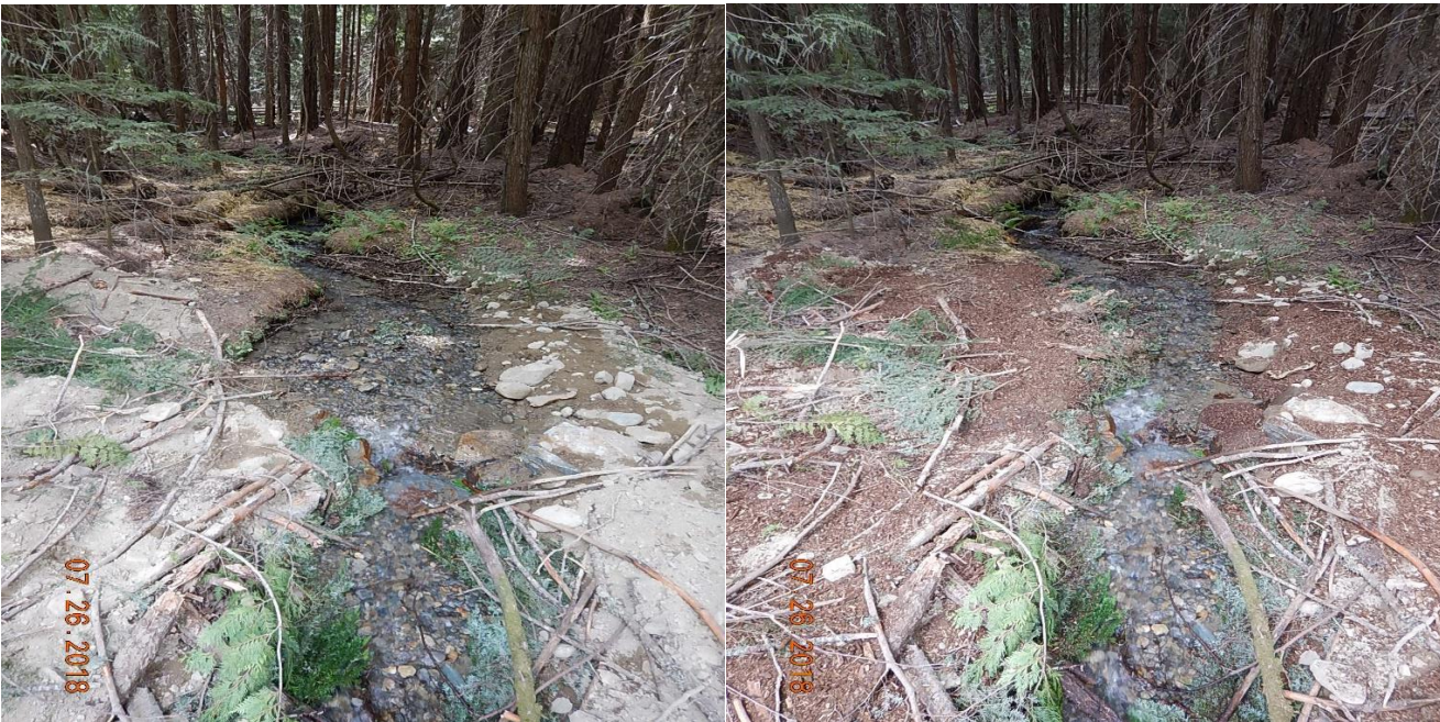
Figure 4: Spring Creek tributary before (left) and after (right) AOP replacement.
