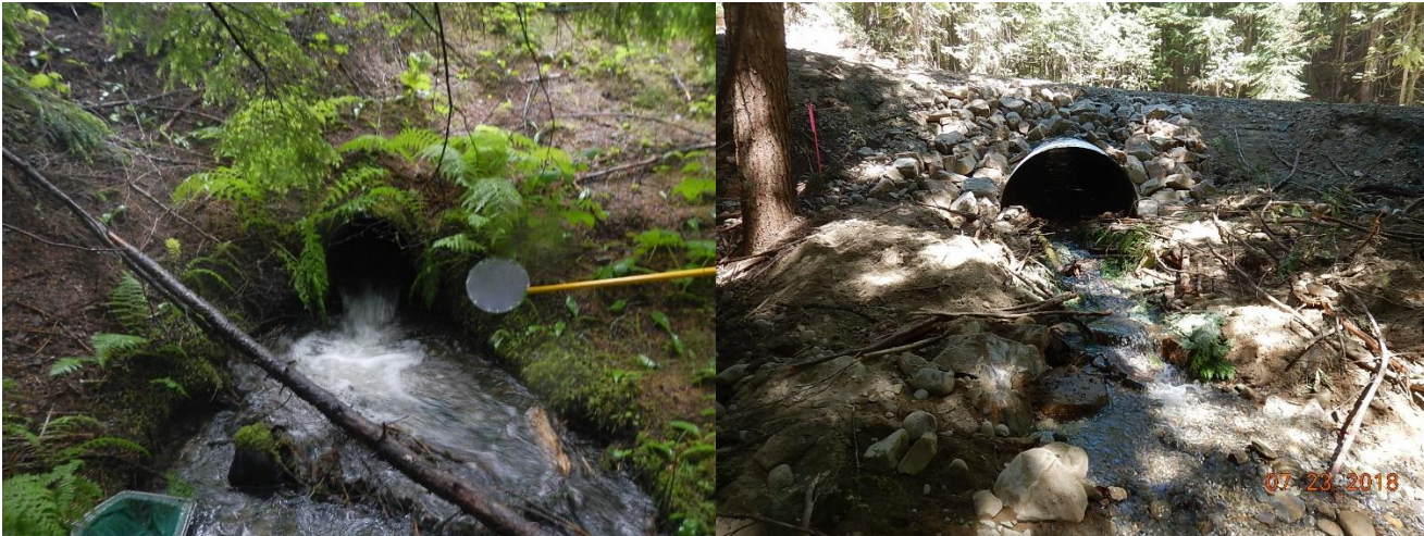
Figure 3: Spring Creek prior to (left) and after (right) AOP replacement.
