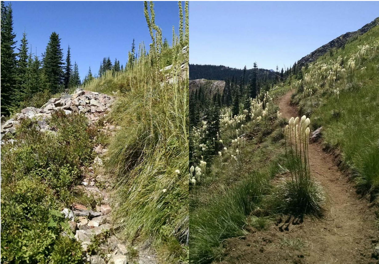
Figure 4: These before and after Slate Ridge trail pictures show traditional trail reconstruction and maintenance work on the district, again using a combination of Forest Service Trail crew and Partners/Volunteers. This highly eroded trail had little soil remaining. The trail tread was re-established to provide better access for multiple users.
