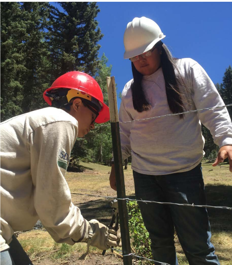
Image 3: Jemez Crew members build fence to protect riparian areas.
