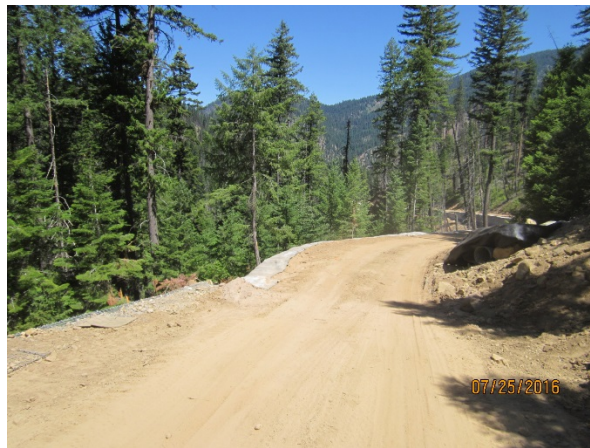
From below – Road Stabilized / Before gravel Surfacing – Long wall
