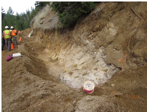
Some existing bedrock needs drilled and blasted / Teaming with Forest Service blasters
