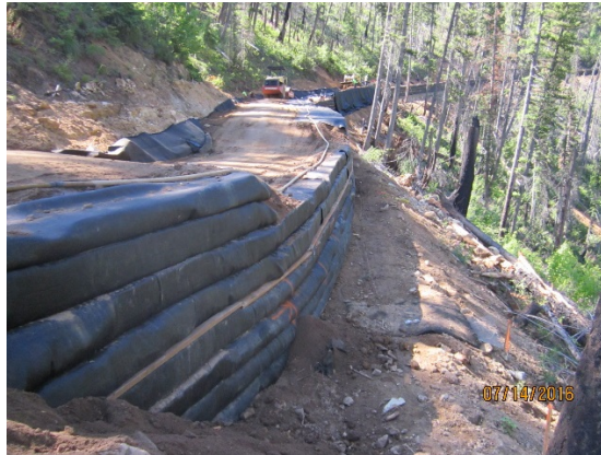
Gabions incorporated in re-design to further stabilize weak slopes / Goesynthetic reinforced soil lifts.
