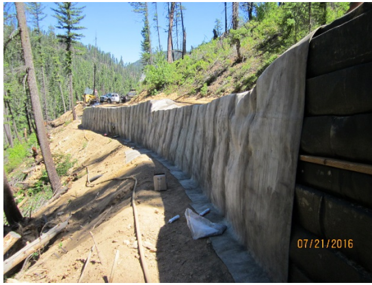
Concrete cloth facing for fire/UV protection.
