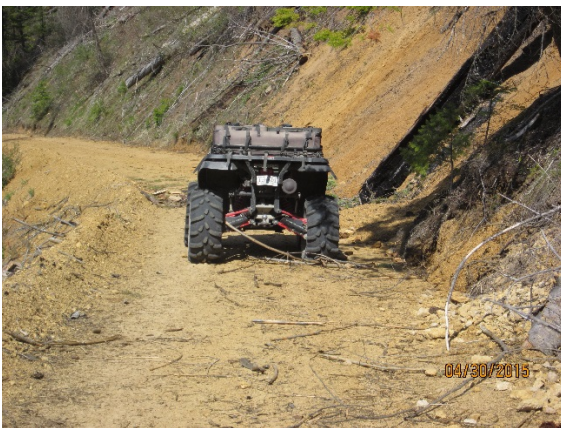
Narrow Road width / Sloughing Cut slope
