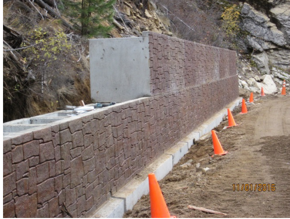
Placing Blocks to lines and grade / Wall construction in progress
