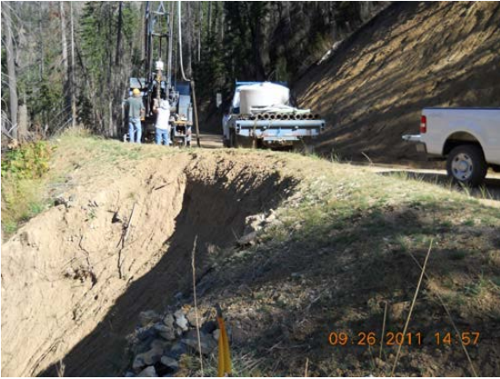
Failed Fill Slope / Fill slope Slide
