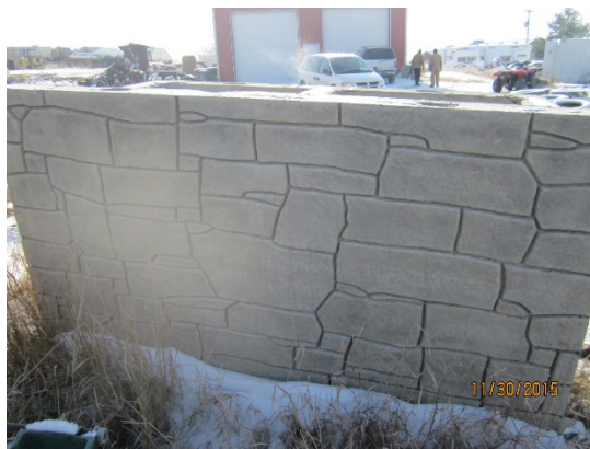
Forms custom built and blocks cast throughout winter months
