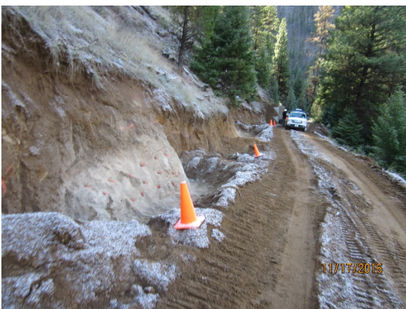
Some existing bedrock needs drilled and blasted / Teaming with Forest Service blasters
