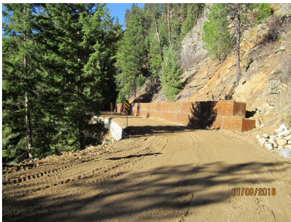
Placing Blocks to lines and grade / Wall construction in progress
