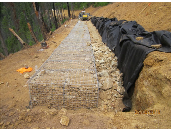
Gabions incorporated in re-design to further stabilize weak slopes / Goesynthetic reinforced soil lifts.
