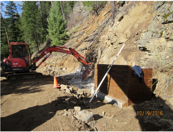
Placing Blocks to lines and grade / Wall construction in progress
