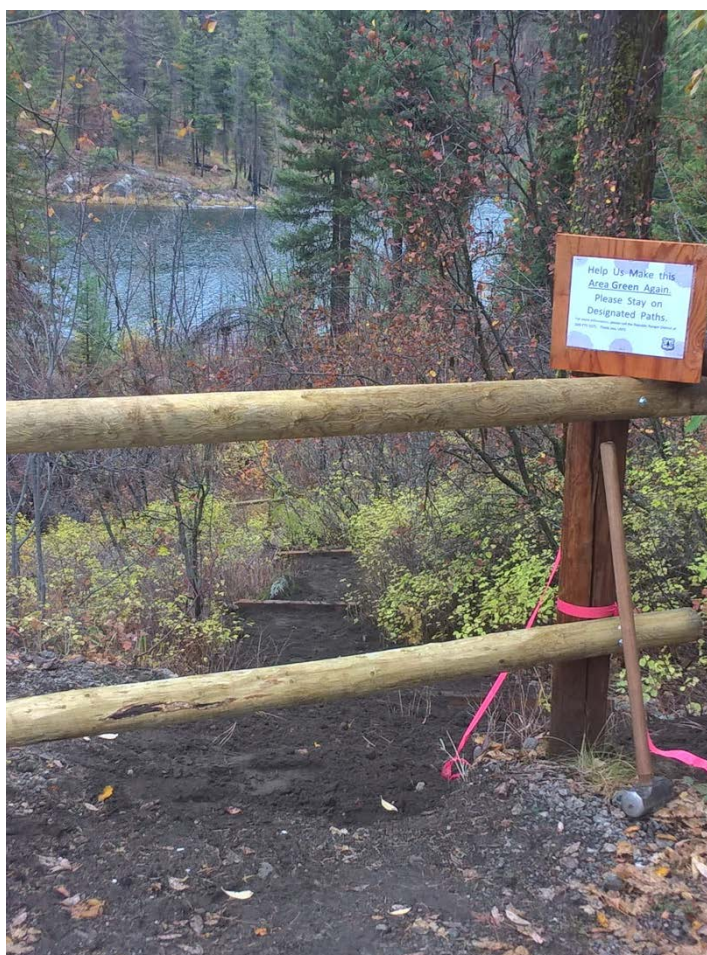
Figure 10. Check dams were installed to define the swim beach and reduce beach erosion. The topsoil in the check dams will facilitate revegetation.
