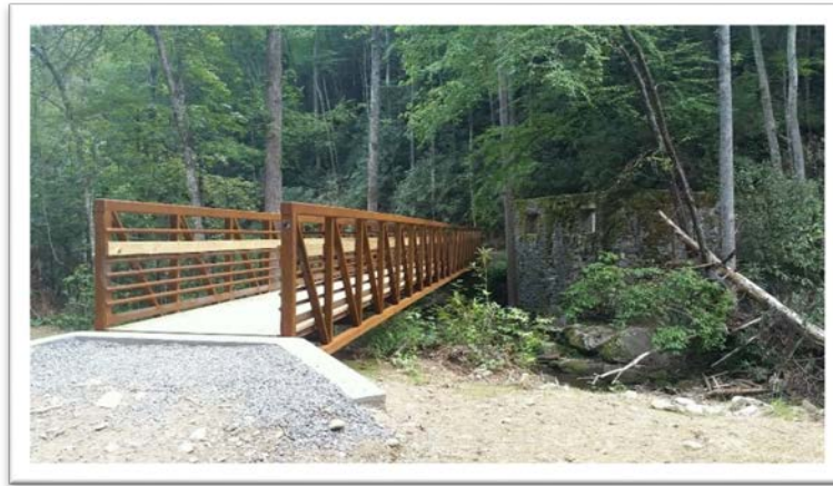
Bridge over Catawba River
