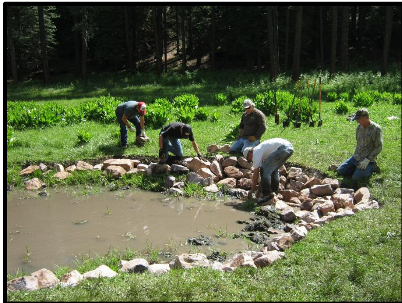
Volunteers build a Zuni bowl in Merritt Draw on the Mogollon Rim Ranger District, Coconino National Forest
