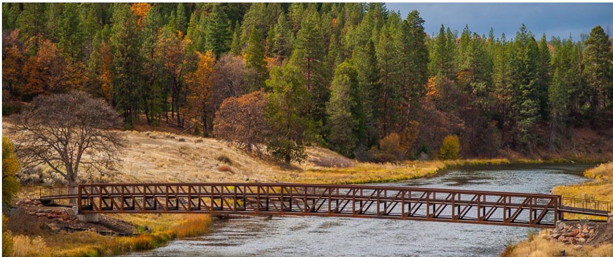
Photo 1- Carbon Bridge (Photo by Val Atkinson)
