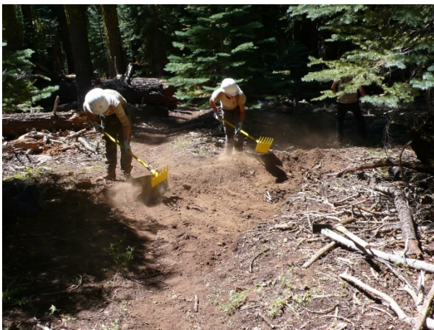
ACE crew members pulling back soil to create rolling dip. Photo by USFS
