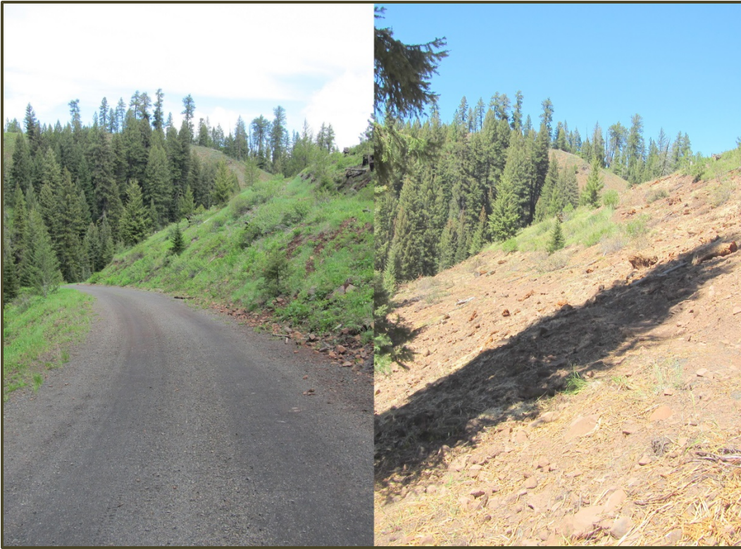
Before and After photos of Road Decommissioning in Dewey Creek
