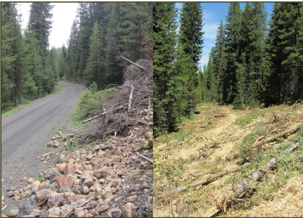
Before and After photos of Road Decommissioning in Dewey Creek
