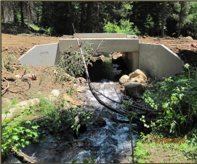
After photos of an Aquatic Organism Passage construction at Ant Basin Creek
