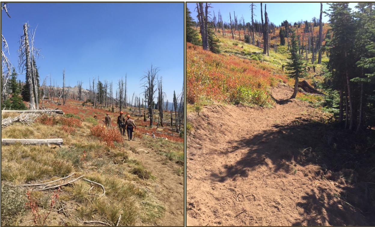
Northwest Youth Corp Working on the Bear Pete Trail Reconstruction
