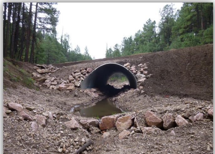
Aquatic Passage Installation
