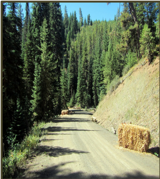
BEFORE: Road Decommission in Joker Creek
