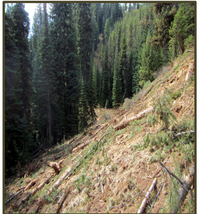
AFTER: Road Decommission in Joker Creek
