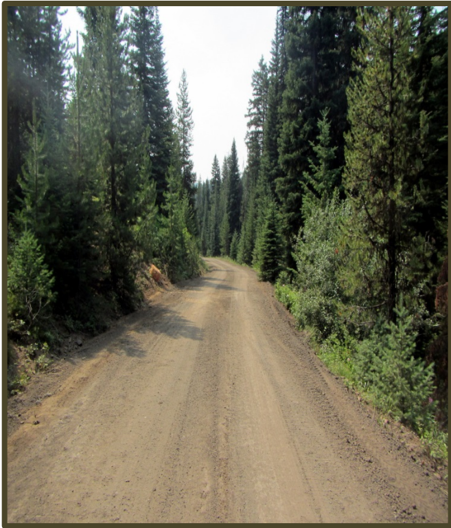
BEFORE: Road Decommission in Joker Creek
