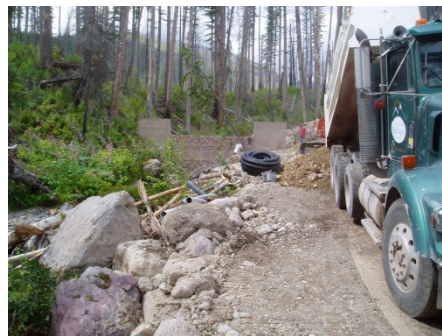
Figure 9: Local contractor during construction.
