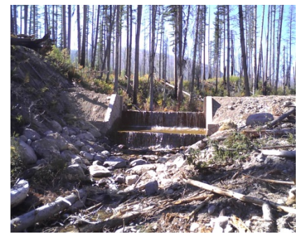
Figure 7: Immediately after construction
