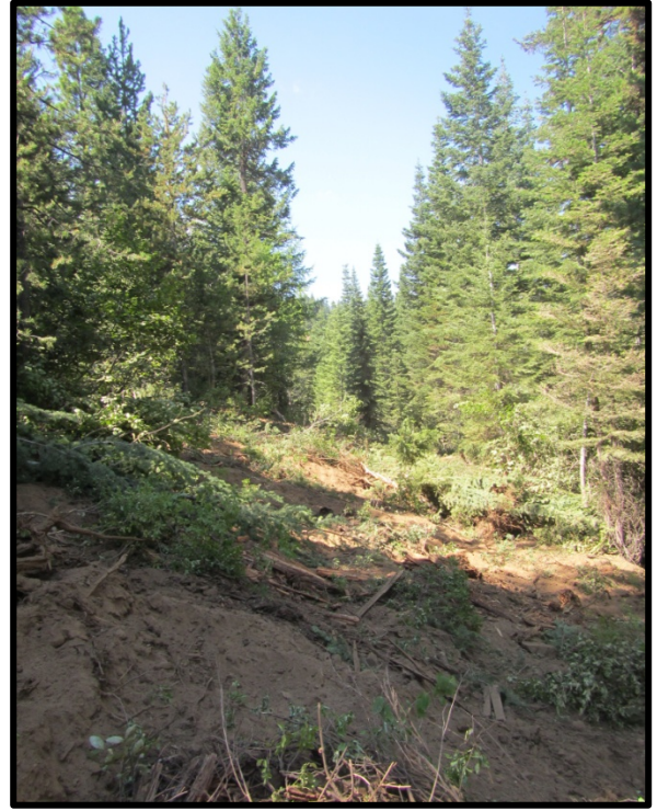
Mill Creek-Council Mountain Project—After
