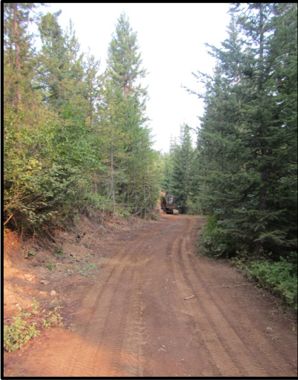
Mill Creek-Council Mountain Project—Before
