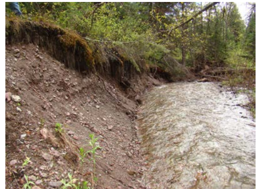
Figure 5: Example of Cottonwood Creek’s current condition, which the Big Blackfoot Chapter of Trout Unlimited is partnering to restore.
