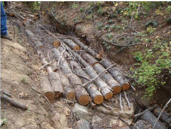
Figure 5 Picture of log mattresses used to repair post fire gullies
