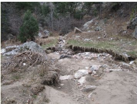
Young's Gulch trail damaged by flooding
