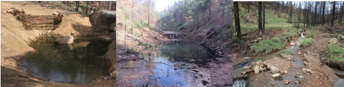
Detention Basin Wellington Gulch Pre-Summer flooding
