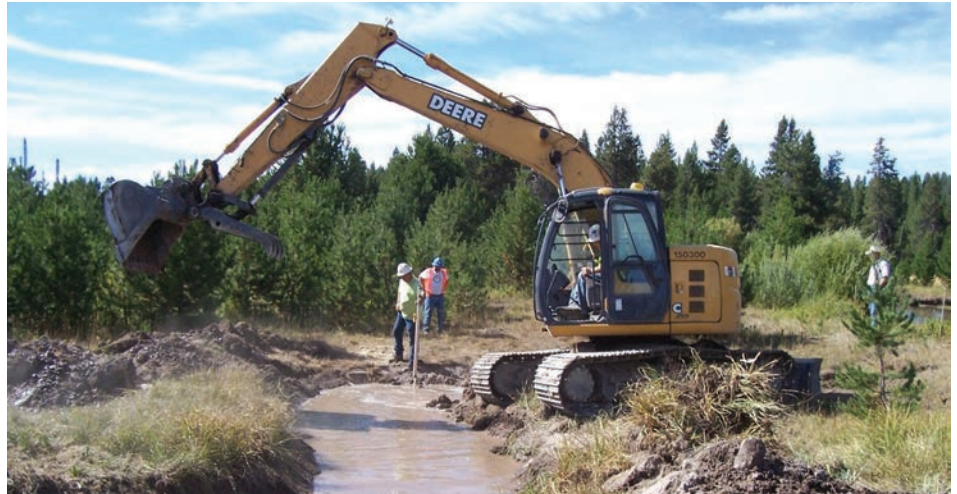
Rebuilding a stream channel to restore connectivity for bull trout, made possible by CFLR. © Craig Bienz
