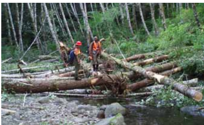
Stream restoration on Hyas Creek, tributary to the Sitkum River in the Quileute's ceded area. The Forest Service and Quileute Tribe cooperated on this project, which involved placing trees, large woody debris, in Hyas Creek to improve fish habitat. Image: Olympic National Forest.
