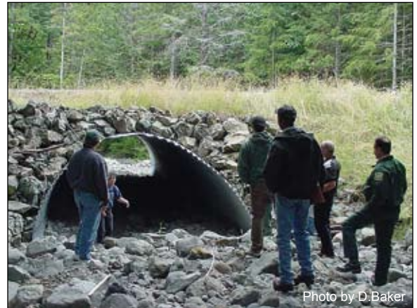
In-stream structure (culvert) to abate seasonal instream passage problem, Olympic Province.
