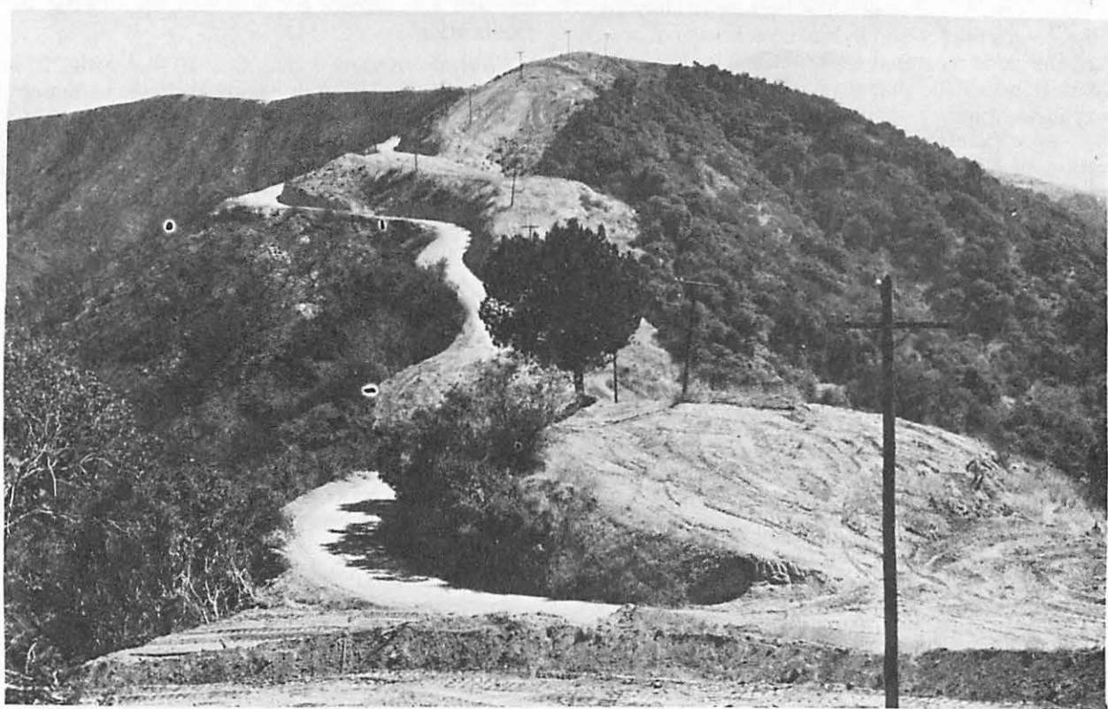
F-523546, 523547 Figure 1.—A fuelbreak (top), usually 200 to 300 feet wide, is vegetated in contrast to a firebreak (bottom), which is generally much narrower, and from which vegetation is cleared each year, or as needed.
