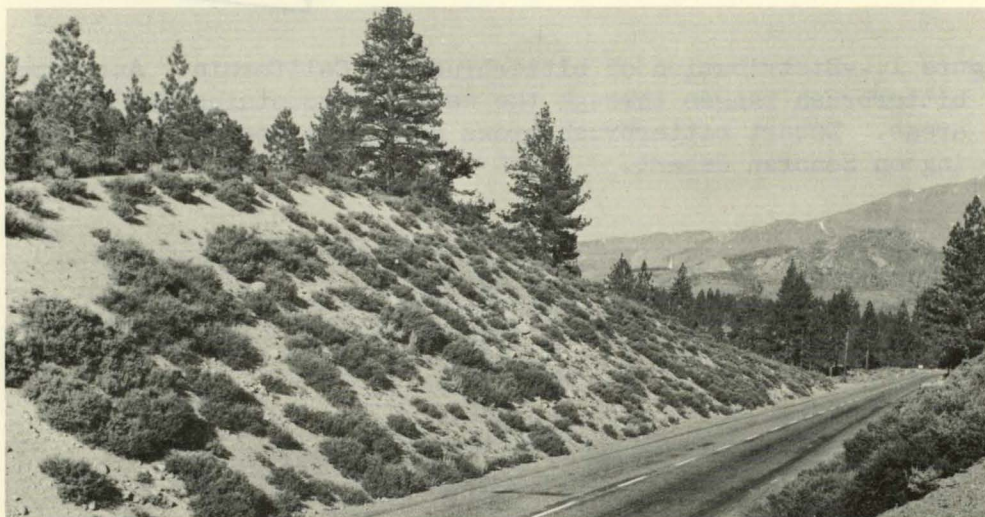
Figure 4.--Road cut stabilized by bitterbrush plants.
