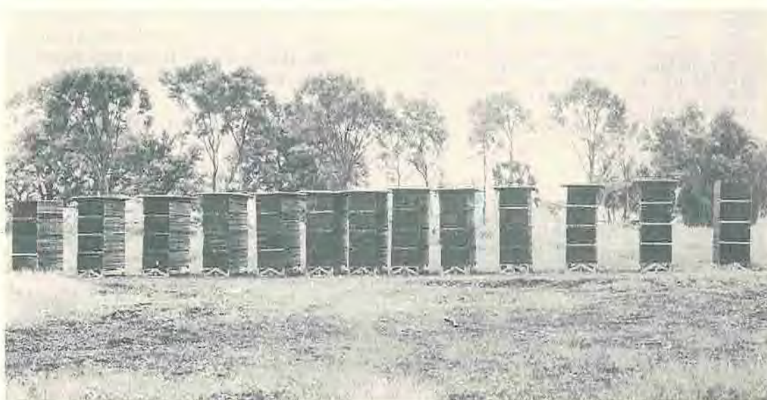
Figure 1. Piles set at increasing spacing, 2 to 6 feet.
