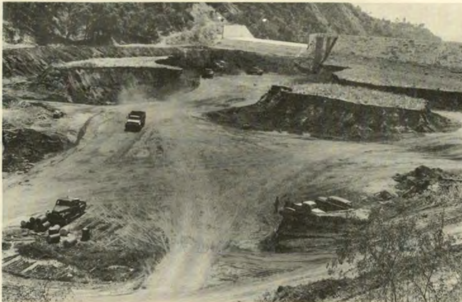
↑ Figure 1.--Material deposited in a debris basin during the rainy season of 1961-62 is removed to maintain storage capacity.
