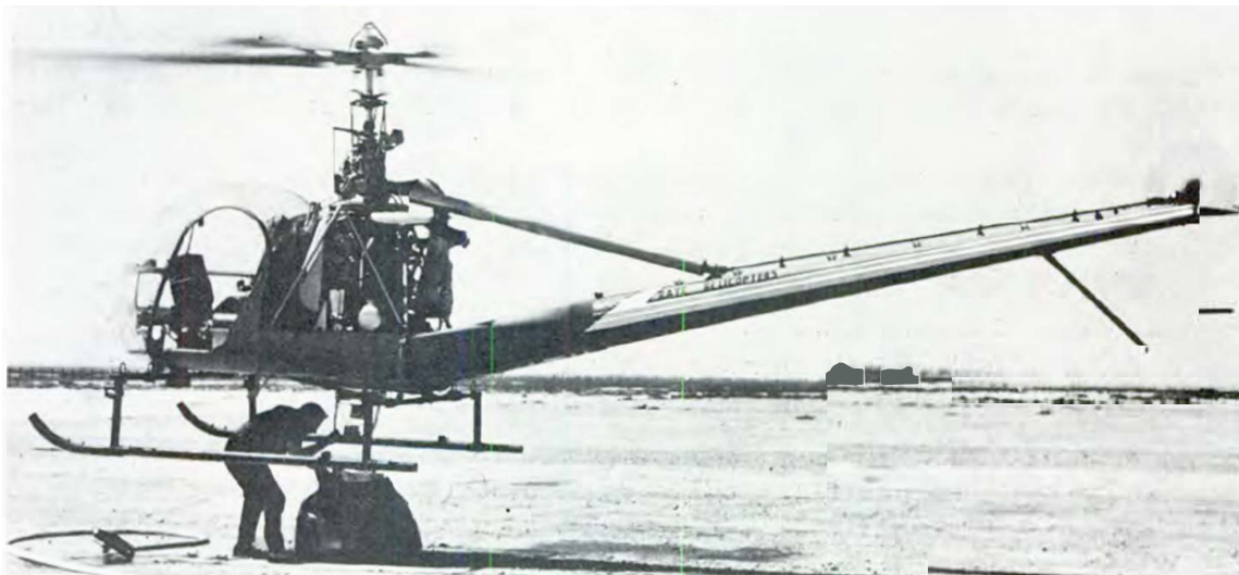
Figure 5.--Filling the Irvin Air Chute tank as it is hovering—or why fire safety officers get grey.
