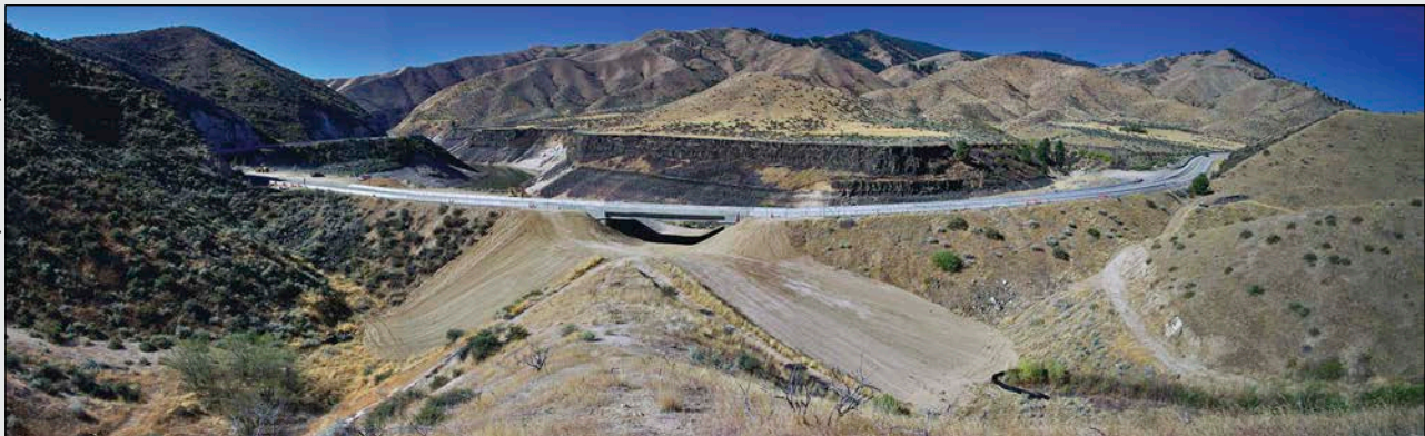
Figure 3— Idaho State 21 wildlife underpass.
