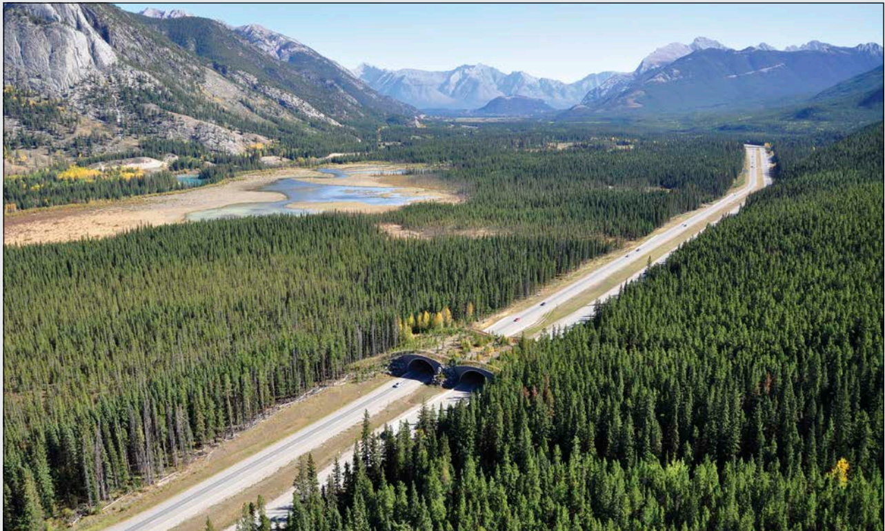
Figure 6—The Wolverine Overpass on the Trans-Canada Highway in Banff National Park, part of the most studied series of wildlife crossing structures in the world.
