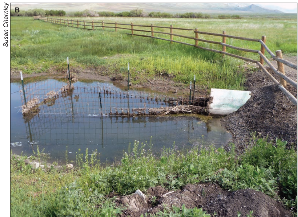
Figure 11—Some ranchers have begun to install devices that help mitigate the negative impacts of beaver: (A) A flow device on the Winecup Gamble Ranch prevents beaver from blocking water flowing under a bridge and flooding a road crossing; (B) A “beaver deceiver” prevents beavers from blocking a road culvert.
