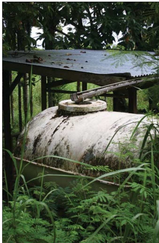
Rainwater collectors, like this one in Saipan, are important for those times when there is insufficient ground water. Photo by Tropical.pete, Flickr.
