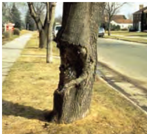
Figure 5.25. This tree has a canker and associated decay that affects >40 percent of the tree's circumference. This tree does not meet safe shell requirements and should be removed.
