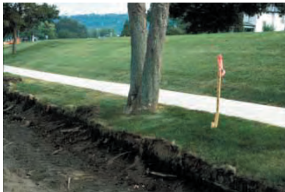
Figure 3.7. When the roots, stem, or branches are defective, a tree can become hazardous.
