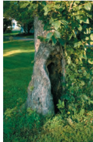
Figure 3.42. High risk of failure: Advanced decay affects more than 40 percent of the stem circumference.
