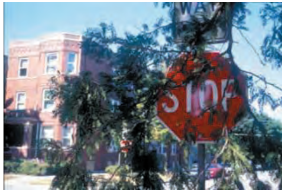
Figure 5.8. Remove all branches that obstruct street signs, signals, street or security lighting or that limit visibility of approaching traffic.
