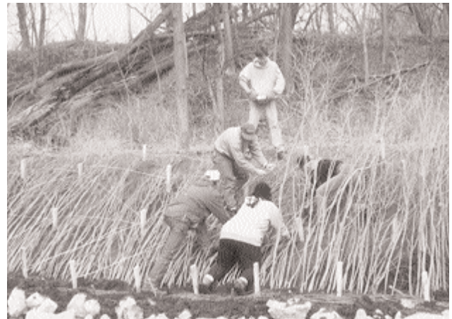
Installing a brushmattress, one of many biotechnical techniques.
