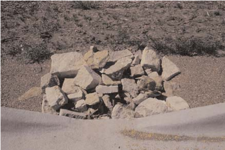
Rocks, located at curb cuts, reduce runoff velocity and energy from the parking lot.
