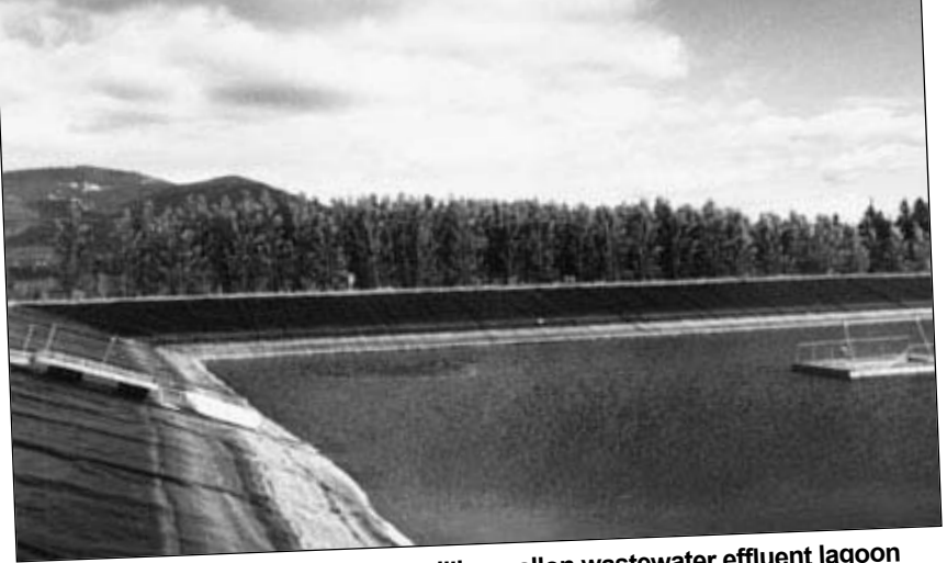
Nine-million-gallon wastewater effluent lagoon with established trees along side.
