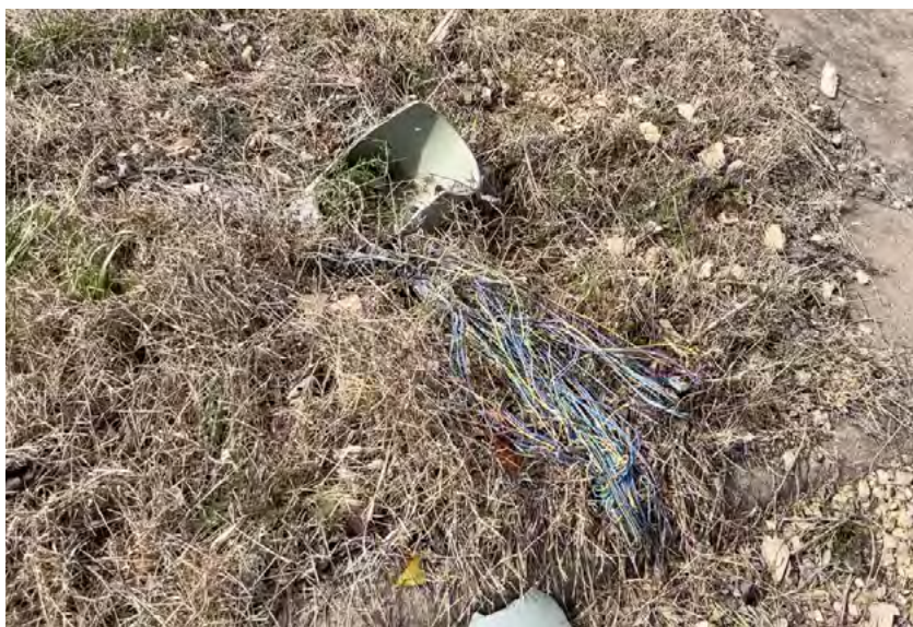
An example of some of the potentially dangerous hidden utilities to look out for before beginning an urban agroforestry project. Photo: Katherine Favor, NCAT
