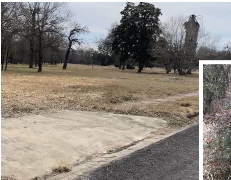
Driveway aprons in need of removal after a buyout demolition in the Upper Onion Creek floodplain.
