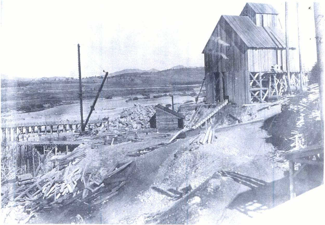
Figure 33. Picture taken sixty days after picture (Figure 32), showing Cement Mill nearly completed. Courtesy of William Balderston.
