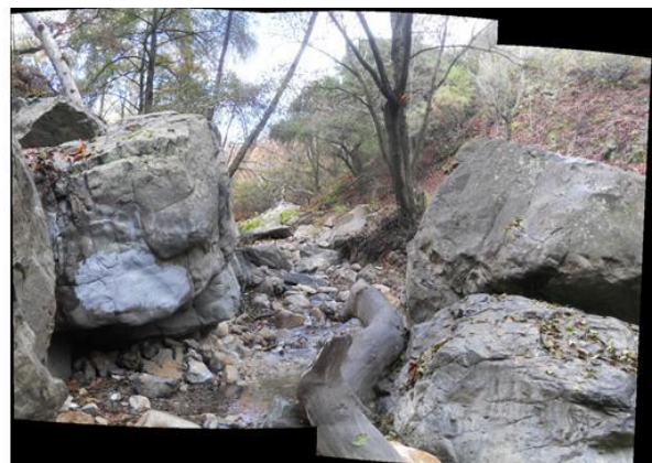
Downstream of dam after demo 19 Dec 2014
