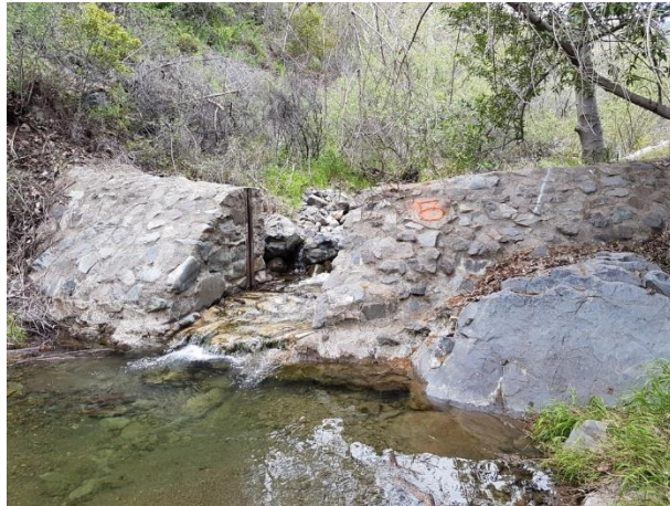
Looking U/S before demo March 2017
