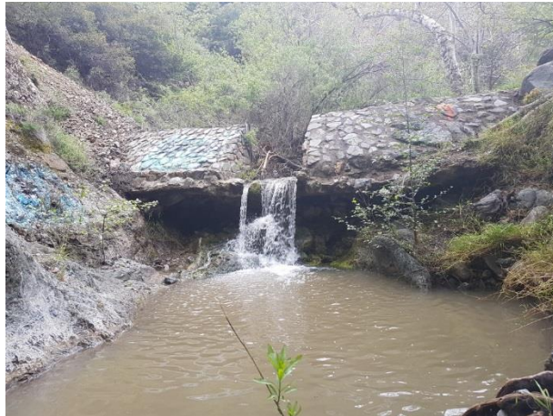
Looking U/S before demo March 2017
