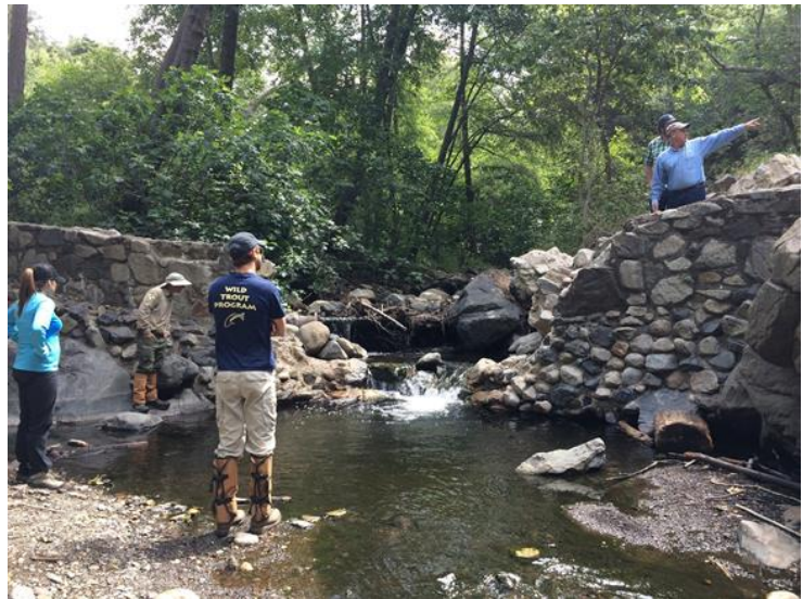
Downstream of dam – May 2017
