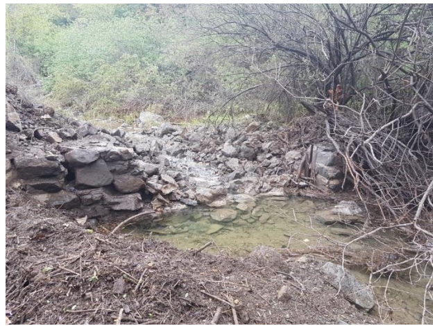
Looking U/S directly after demo March 2017
