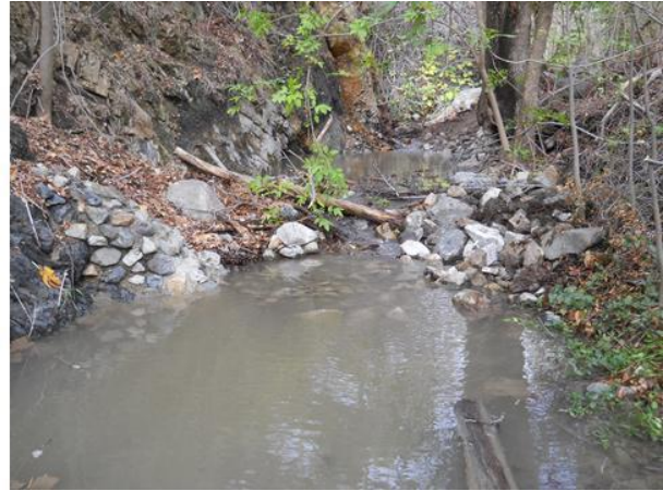
Downstream after demo 19 Dec 2014
