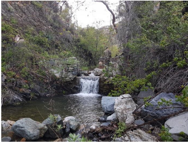
Looking U/S before demo March 2017.
