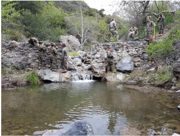
Looking U/S before demo March 2017
