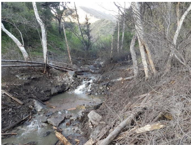
Looking U/S directly after demo March 2017
