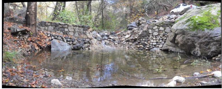
Downstream of dam after demo 19 Dec 2014
