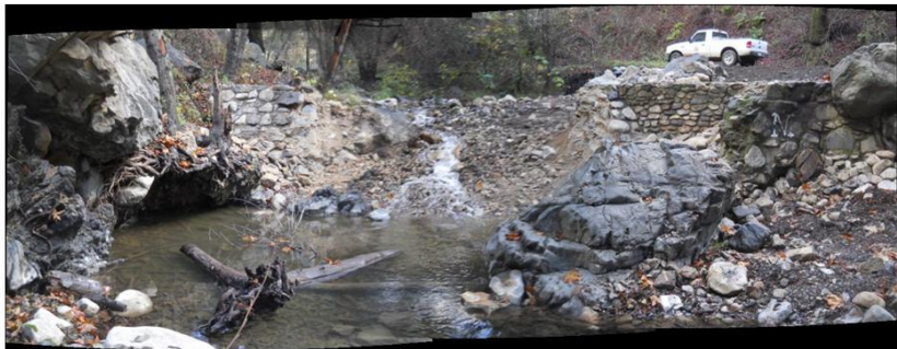
Downstream of dam after demo 19 Dec 2014
