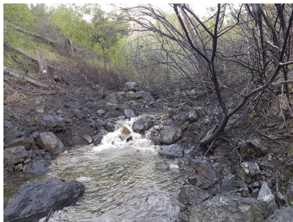
Looking U/S directly after demo March 2017
