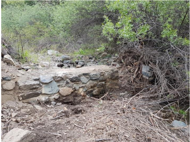
Looking U/S before demo March 2017
