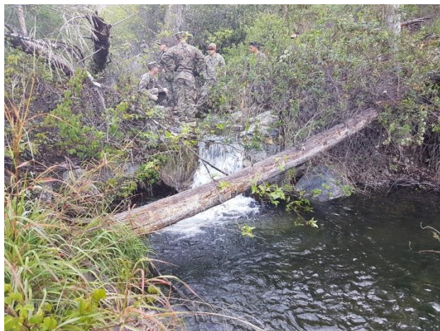
Looking U/S before demo March 2017
