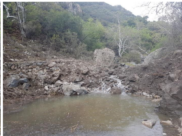
Looking U/S directly after demo March 2017
