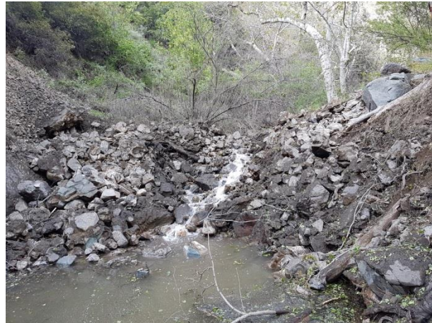
Looking U/S directly after demo March 2017
