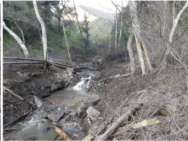
Looking U/S directly after demo March 2017
