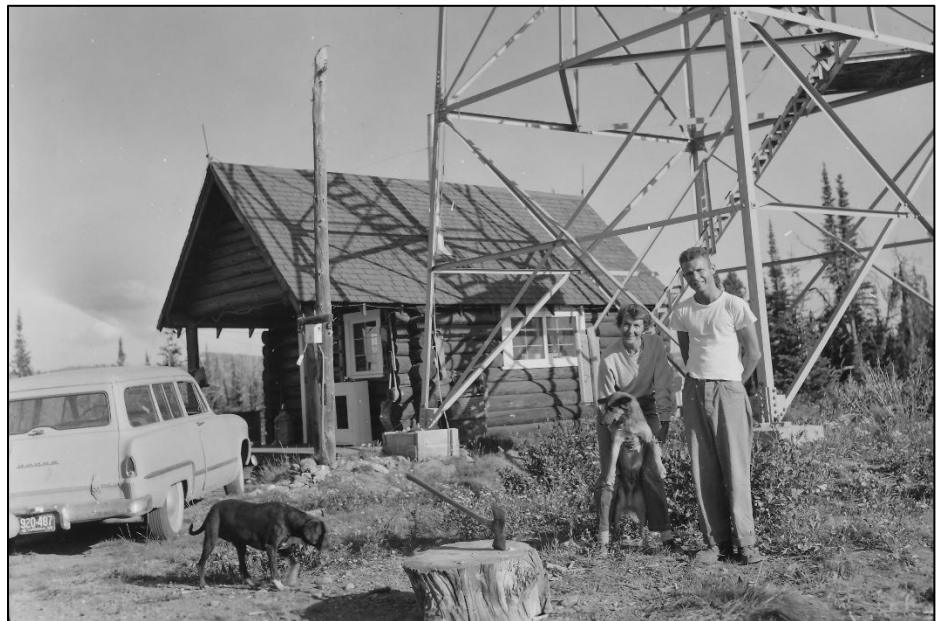
Carey Dome cabin and lookout, post-1943.
