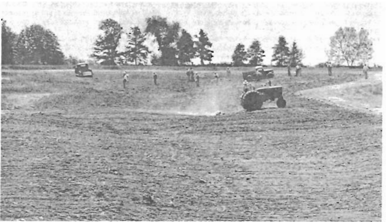
Figure 8.--Above, gully near Berryville, Ark., before rehabilitation. Below, gully leveled and filled, ready for sodding.
