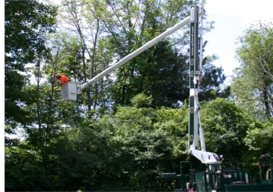
Tree removal (H. Liu, Pennsylvania DCNR)
