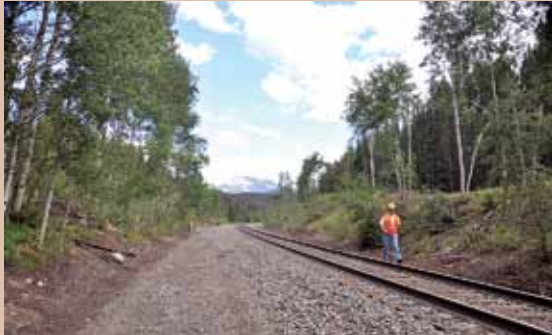
Winter Park cleared beetle-killed trees from 3.1 miles of railroad easement. Top photo, before treatment. Bottom photo, after treatment. (Photos by Kathryn Hardgrave)
