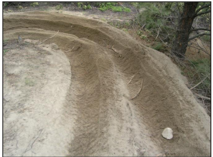
Figure 90—Loop D turn, rut depth 10 inches.
