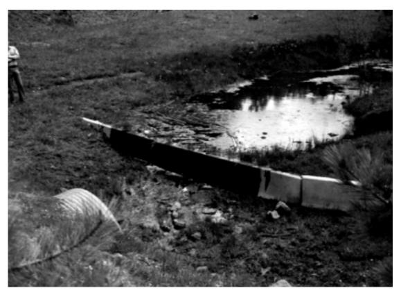
Figure 3—Jersey barrier gully plug.
