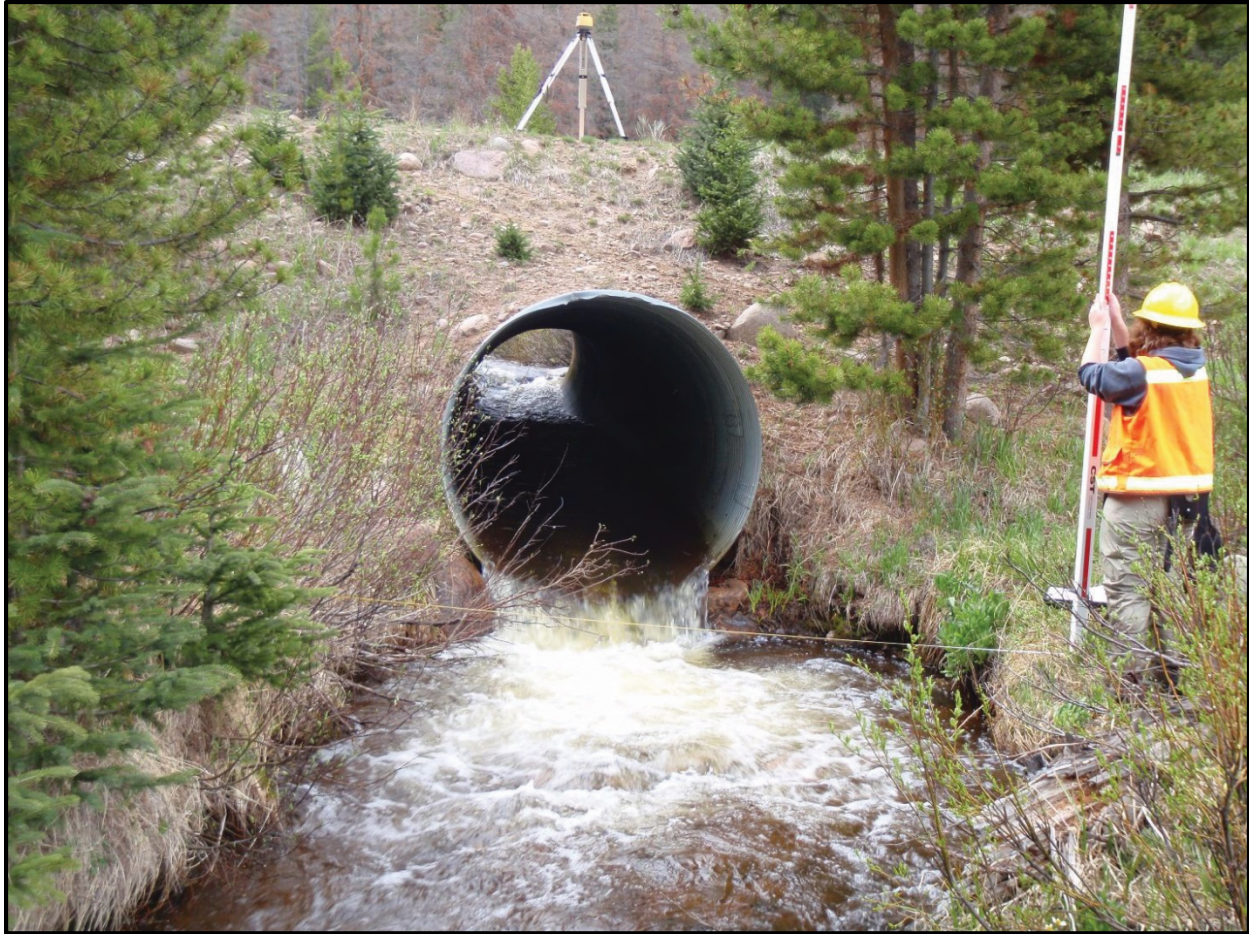
Figure 3. A road-stream crossing that does not mimic natural stream reaches, but may still allow AOP for certain species. A Level-1 physical assessment should be conducted.
