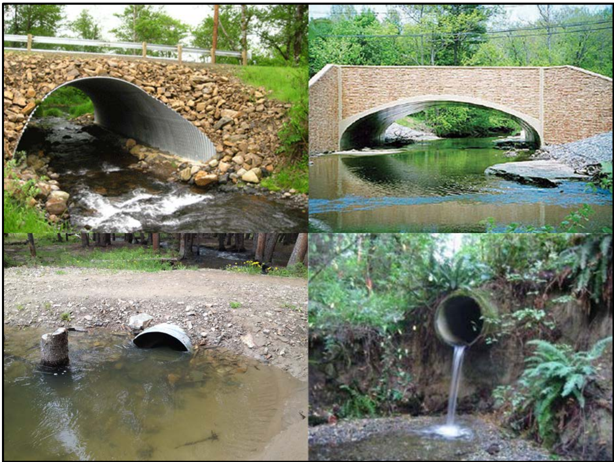
Figure 4. Pictures in the upper two panels depict road-stream crossings that could be considered to mimic natural stream conditions, while the two lower pictures show crossings that clearly do not meet those criteria. The top two culverts appear to maintain natural stream flow similar to adjacent reaches and contain natural substrate similar to upstream and downstream reaches, whereas the bottom left culvert does not maintain an opening wider than the channel width, and the bottom right culvert has an outlet perch height greater than 150% of that of the outflow pool depth.
