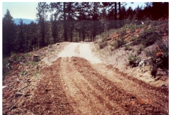
Figure 22. Chipped slash road surfacing absorbs and retains moisture from precipitation events.
