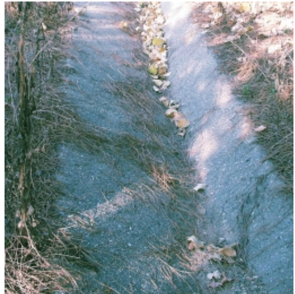
Figure 14. Paved ditch for erosion abatement.
