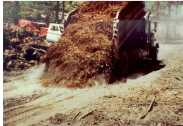
Figure 21. Spreading chipped slash as a lightweight road surfacing.
