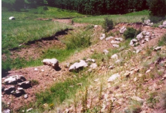
Figure A4. Gully erosion directly downhill of road segments A-B and B-C due to surface water concentration and flow.
