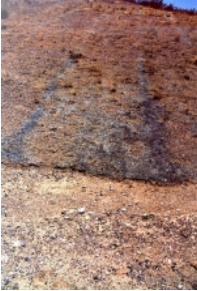
Figure 6. Organic mat back slope erosion abatement.
