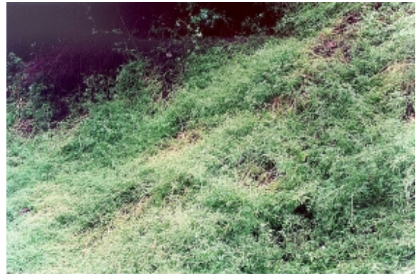
Figure 5. Revegetated fill slope, stable and resistant to erosional processes.
