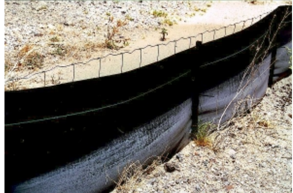
Figure 9. Wire mesh reinforced silt fence.
