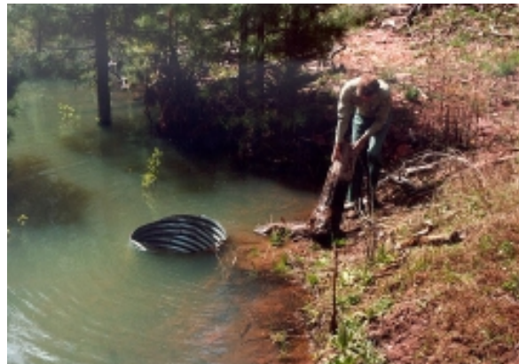
Figure 18. Raised inlets on road stream crossing to pond water and preserve sediment.
