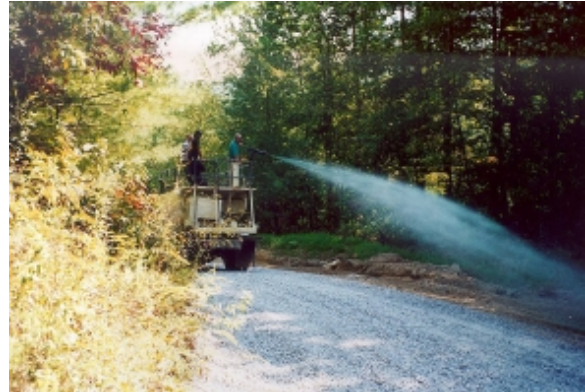
Figure A15. Hydroseeding unsurfaced shoulder of reduced width road.
