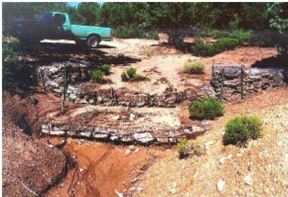
Figure 12. Cross drain outflow armored by gabion structure.
