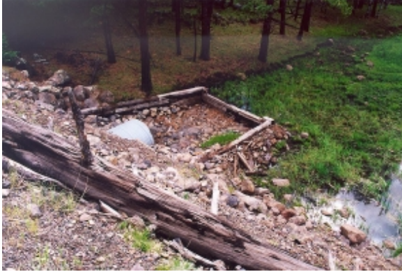
Figure 20. Used railroad tie structure to pond water and preserve sediment upstream of a road stream crossing.
