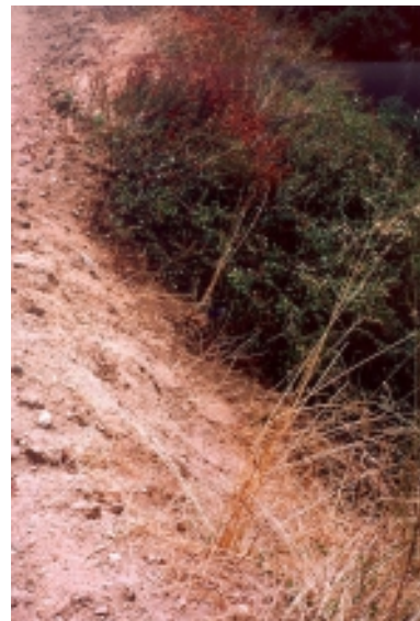
Figure A11. Brush is holding berm on fill slope (top). When brush dies, berm material is available for movement down the hill slope.
