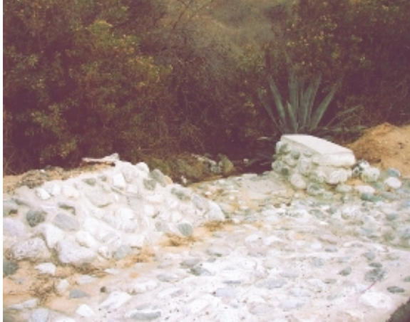
Figure 11. Grouted rock riprap protection for cross drain outflow.
